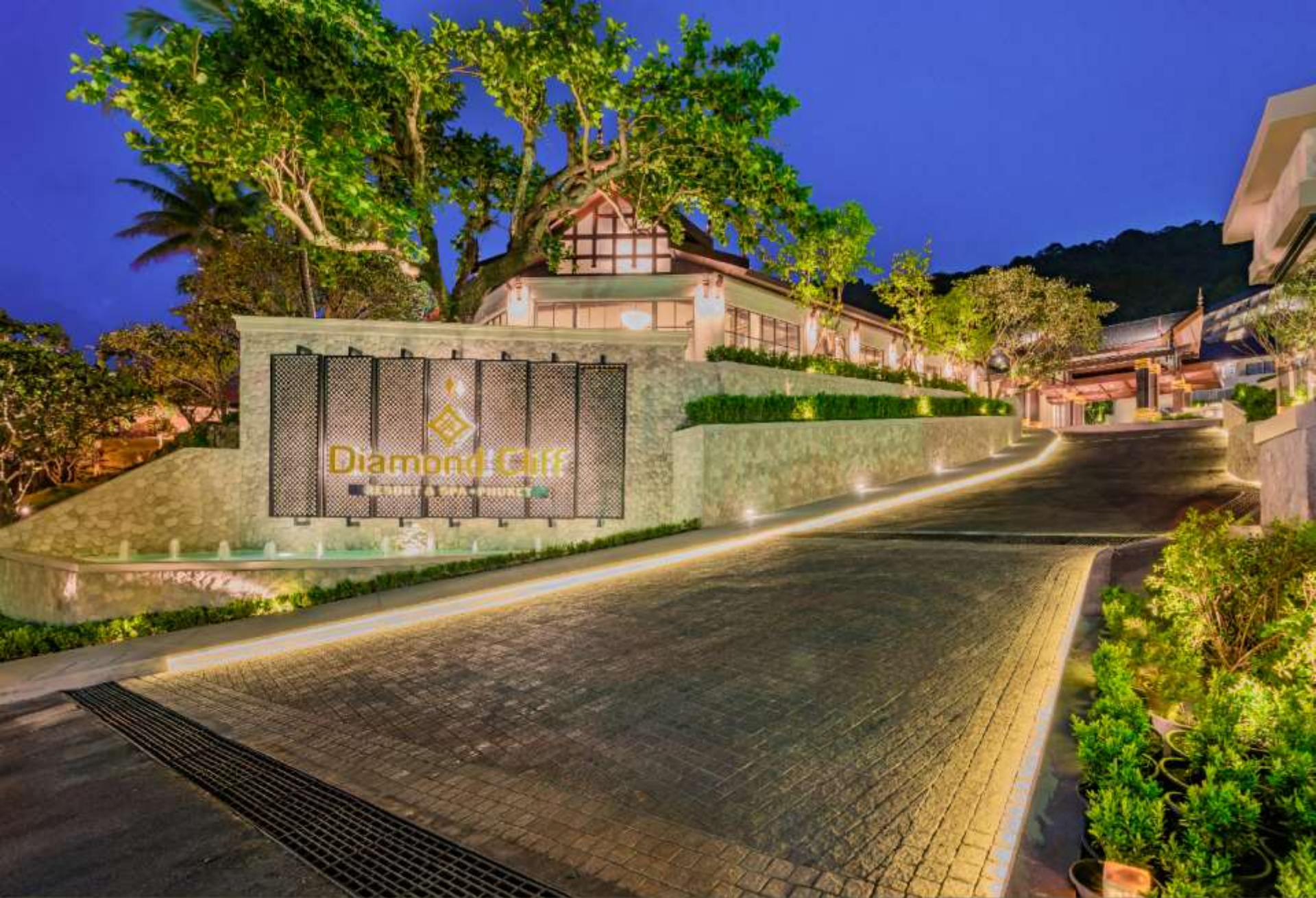
Hotel Main Entrance
